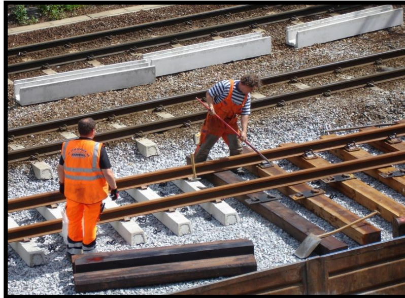
Figure 2-15 Timber transverse sleepers for railway track [5].
