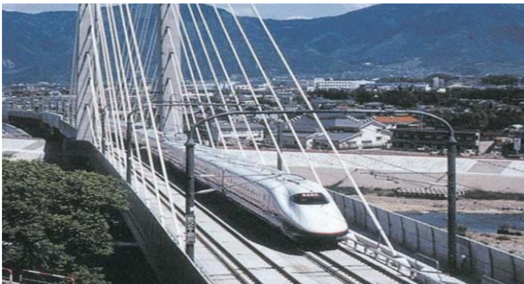
Figure 2-22 Bridge or elevated structure of railway [24].
