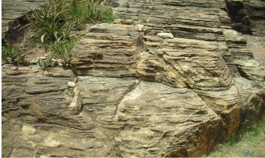
Figure 2-4 thinly bedded and jointed Enticho sandstone
