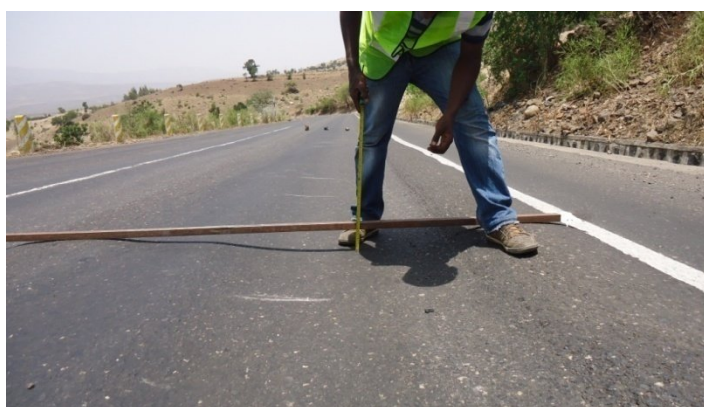
Figure 3-3 Rut depth measurement at section-7 (km 26+800)
