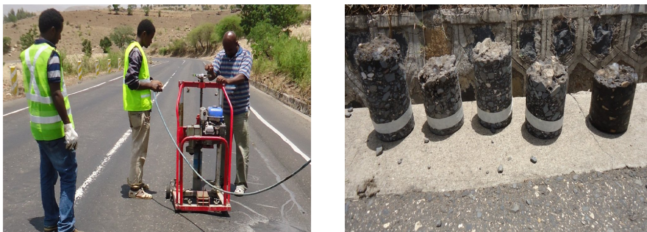
Figure 3-5 Typical core sample extraction process and extracted core samples at km 26+800
