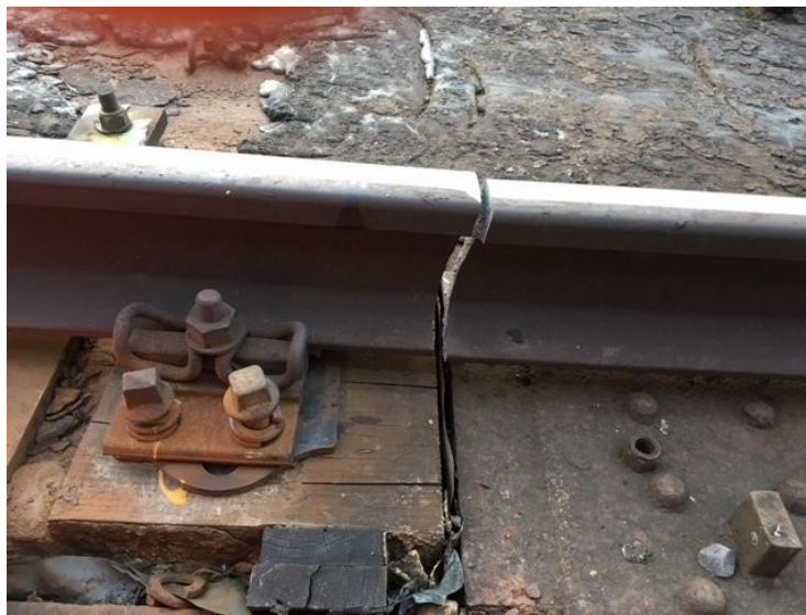
Fig. 2. 3. Broken rail [35]
