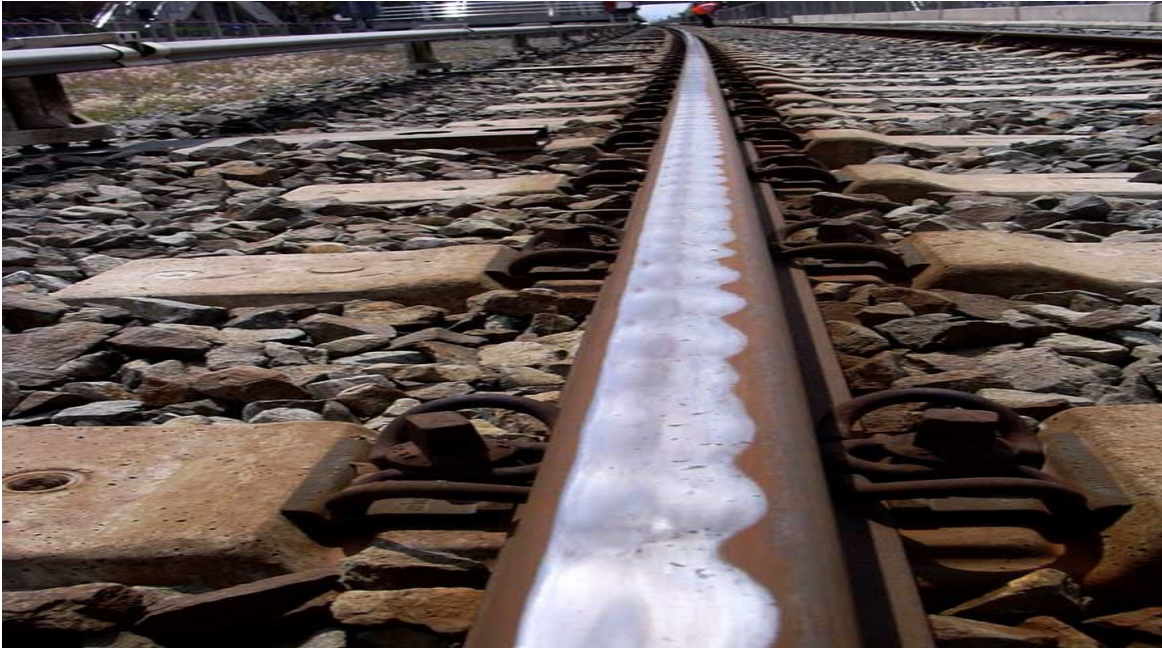
Fig. 1.5. Railway Rail corrugation [14]
