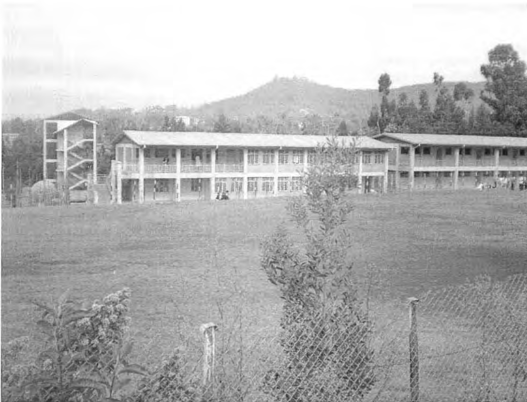
Figure 3. Entoto Amba secondary school
