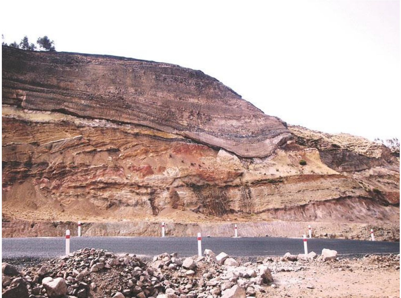
Figure 3-8: The Jima Volcanites at the top of the Guraghe escarpment. Gently inclined rhyolite ignimbrites incised by a channel in turn filled by horizontally laminated ignimbrite flows. New road on the western flank of the MER between Butajira and Welkite shows the existing geological features (Ernesto et al. , 2015).
