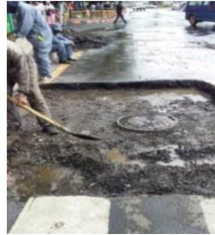
(c) Repair work around manhole
