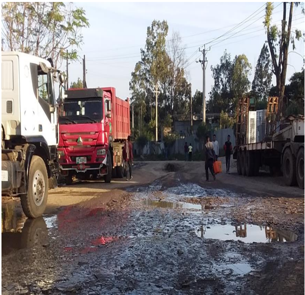
(c) Heavy vehicles over/mis using the road
