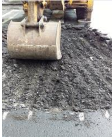
(a) Excavation to asphalt
