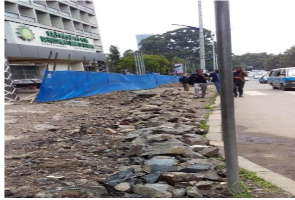
(a) Muddy & inconvenient excavated sidewalk (b) poorly reinstated side walk enforce pedestrians to accidentally share roadway with vehicles
