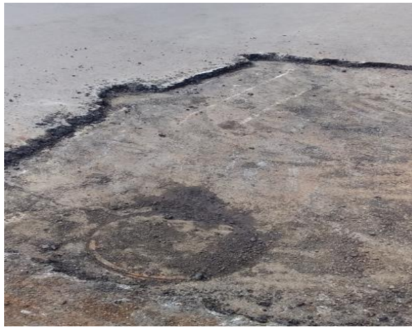
(d) Removal of damaged surface course due to ingressed water
