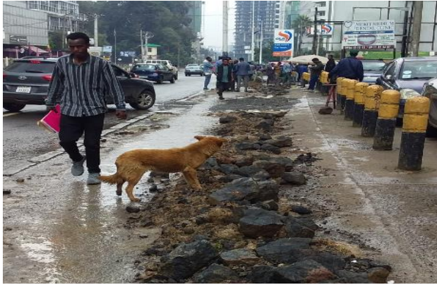
(a) Muddy & inconvenient excavated sidewalk (b) poorly reinstated side walk enforce pedestrians to accidentally share roadway with vehicles
