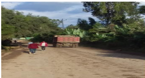
(a) Rough asphalt road surface due to cart away material (b) Muddy asphalt surface due to cart a way
