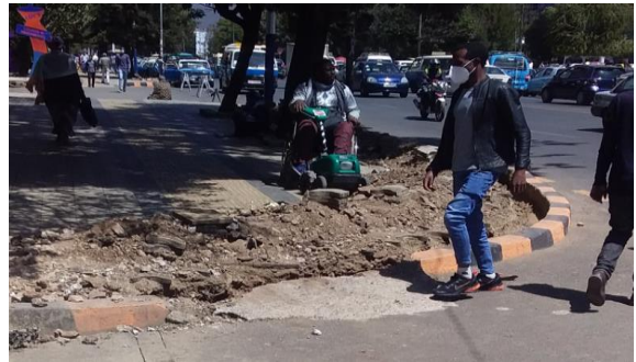
(b) Disabled and wheel chaired man facing trench ahead
