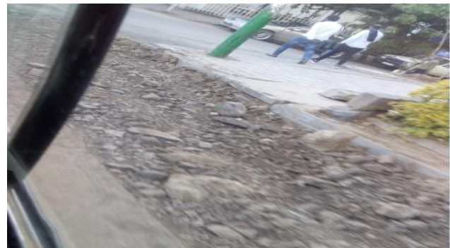
(a) Accidentally shared roadway by pedestrians due to dumped material (b) Poorly reinstated trenched roadway
