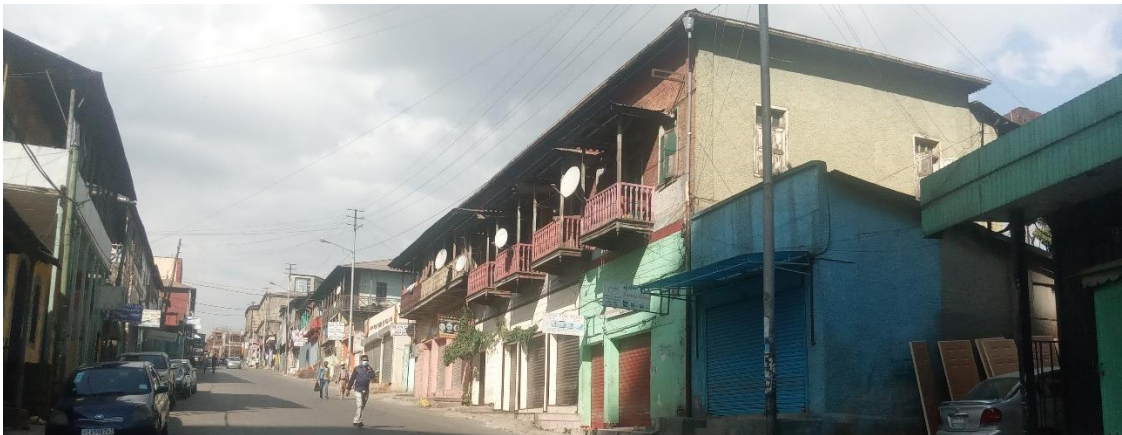
Figure 19 upward view of historic buildings
