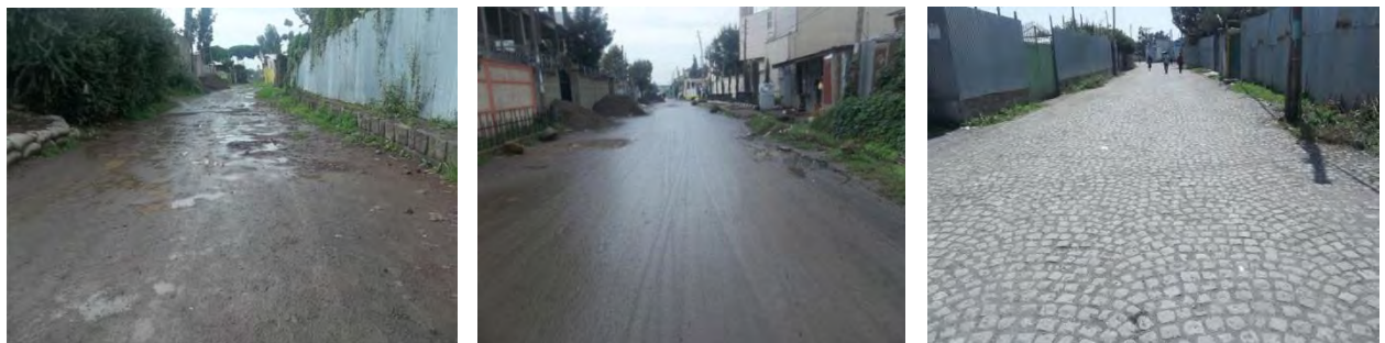
Figure 6. 26 Street pavement types (Earth, Asphalt and cobblestone) Source: Fieldwork (2016)
