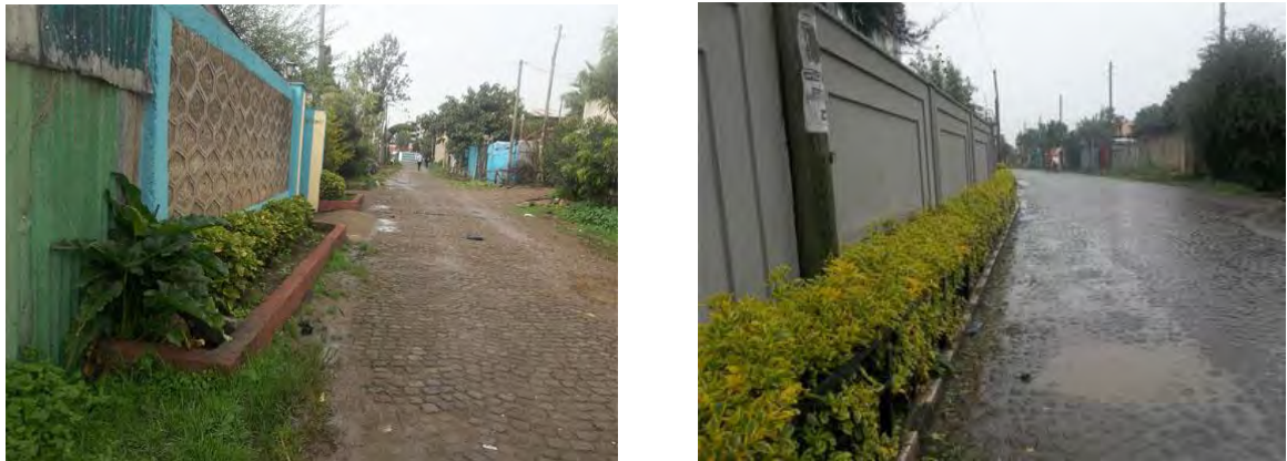
Figure 6. 29 Form of bioretention with curbstone around it with no break in between Source: Fieldwork (2016)
