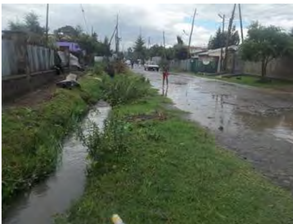
Figure 6. 33 Overflow from the drainage to the streets Source: Fieldwork (2016)
