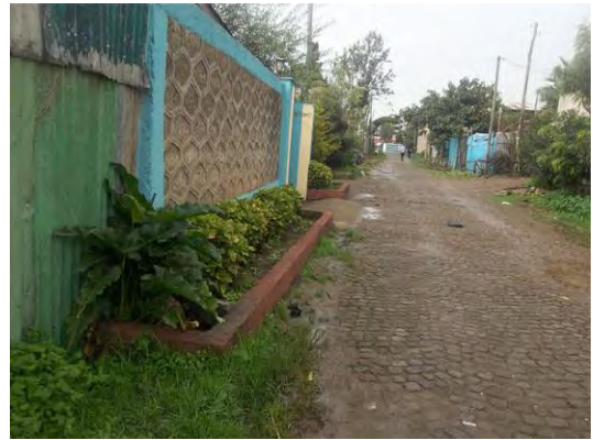
Figure 6. 39 Form of bioretention along the fence Source: Fieldwork (2016)
