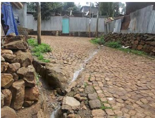
Figure 6. 37 Diagonal street drainage Source: Fieldwork (2016)
