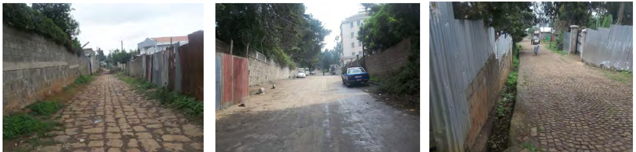
Figure 6. 22 Street pavement types (Stone, Asphalt and cobblestone) Source: Fieldwork (2016)
