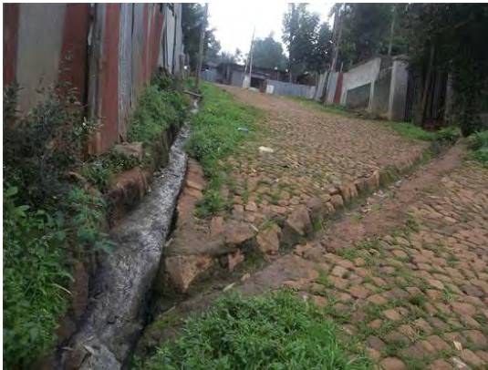
Figure 6. 35 Diagonal street drainage construction Source: Fieldwork (2016)
