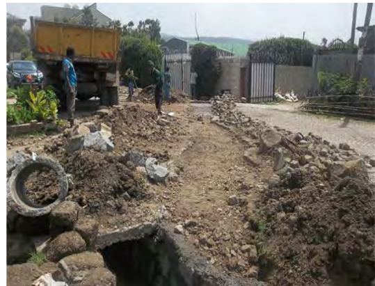
Figure 6. 41 Street drainage construction Source: Fieldwork (2016)
