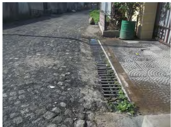
Figure 6. 36 Drain grating cover Source: Fieldwork (2016)
