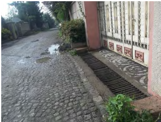
Figure 6. 40 Drain grating cover Source: Fieldwork (2016)
