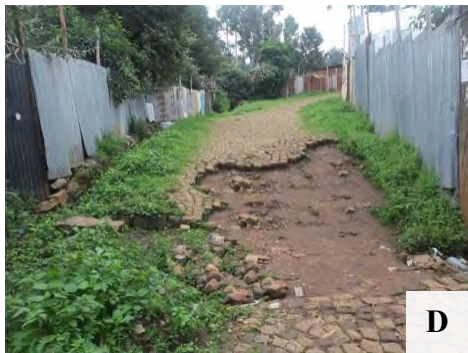
Figure 6. 24 Fragmented cobblestone pavement Source: Fieldwork (2016)
