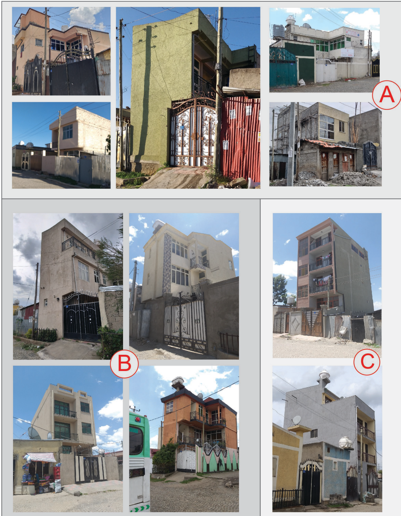
Figure 2011, Multi-storey Building in the 'Mekelakya Sefer', A - G+0, B - G+2, C - G+3 residences
