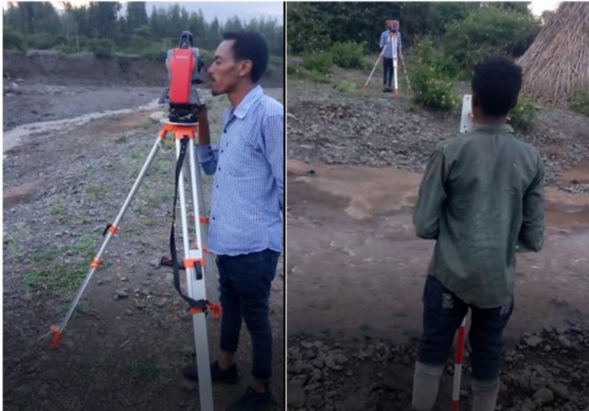
Figure 3-7 River cross section data collection using total station of at April 14, 2019
