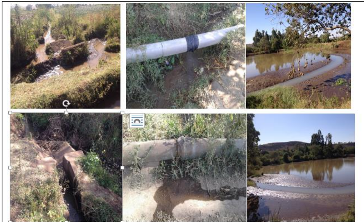
Figure 4.7: Irrigation water conveyance systems damaged canals (left) broken PVC (middle) and pond filled with sediments (right) (Source: own picture 2017).
