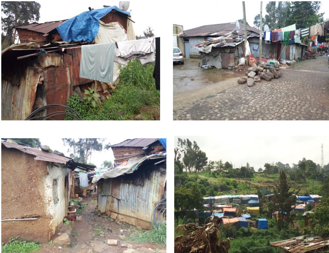
Figure 4.3: Houses in the Study Area a) kebele house with iron corrugated wall in Arada sub city (top left) b) kebele house with low and leaking roof in Addis Ketema sub city (top right) c) congested kebele houses in Arada sub city (bottom left) d) temporary shelter with plastic thatch in Arada sub city (bottom right) (Source: direct observation, 2018)
