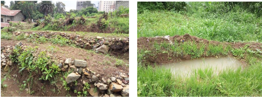
Figure 4.17: Watershed Management Area a) stone bunds and table terraces in Arada sub city (left) b) trench made for reserving water in Arada sub city (right) (Source: direct observation, 2018)
