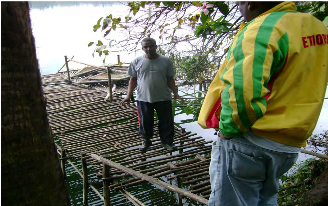
Figure 5: Picture showing the jetty construction and cage anchoring site
