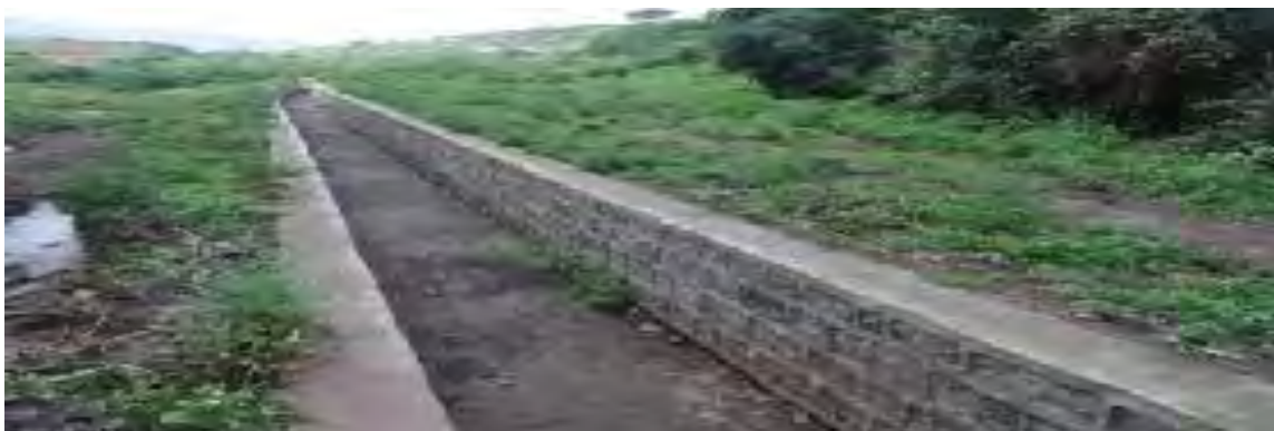
Plate 6. Diverted built-up area runoff
