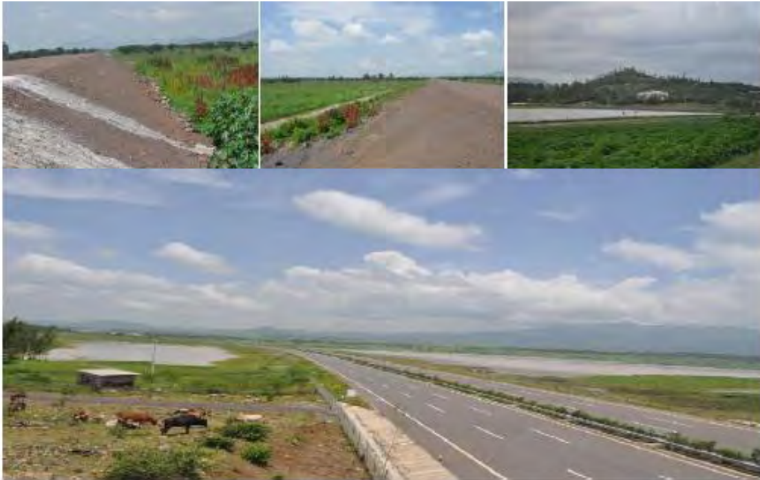
Plate 5. Diverted stream flow
