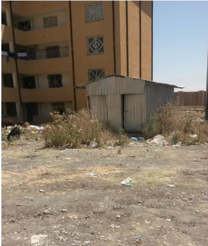
Picture 6: The only latrine in the relocation site (08/03/15)
