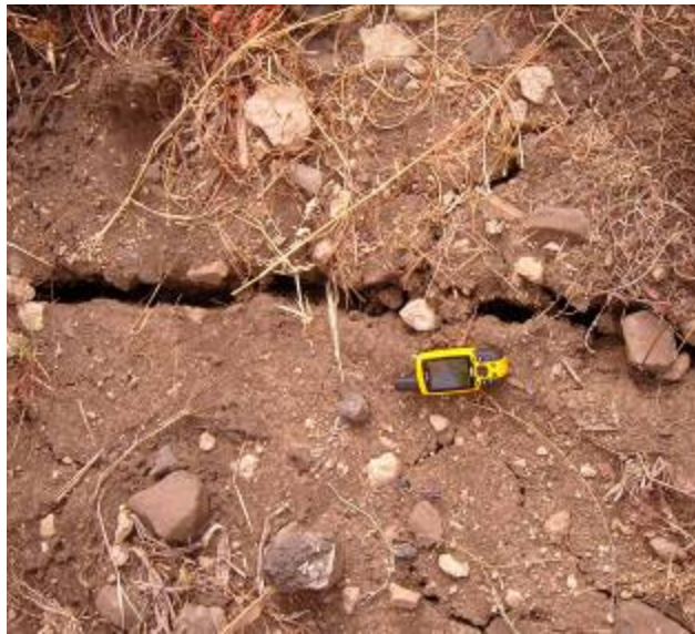
a. Tension crack on agricultural land
