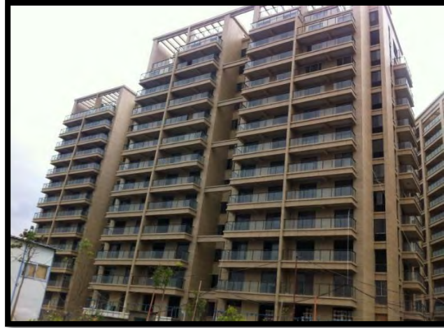
Figure 20: Tsehay real estate G+12 apartment houses
