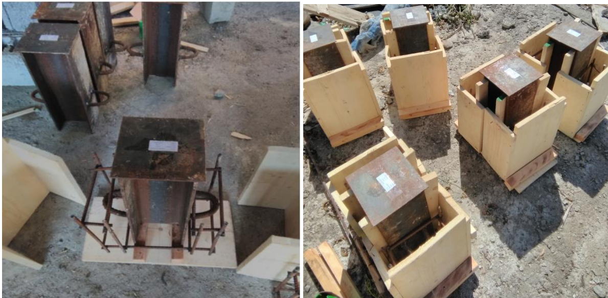
Fig 3.8): formwork preparation for solid concrete
