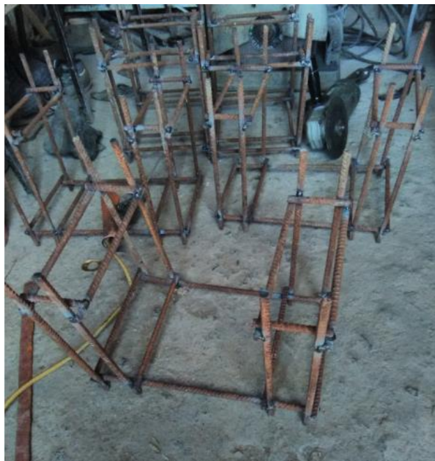
Fig 6.2): 10mm diameter transverse reinforcement welding at intersection
