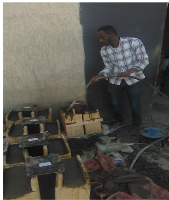
Fig 6.6) pouring and compacting of concrete by using mechanical vibrator
