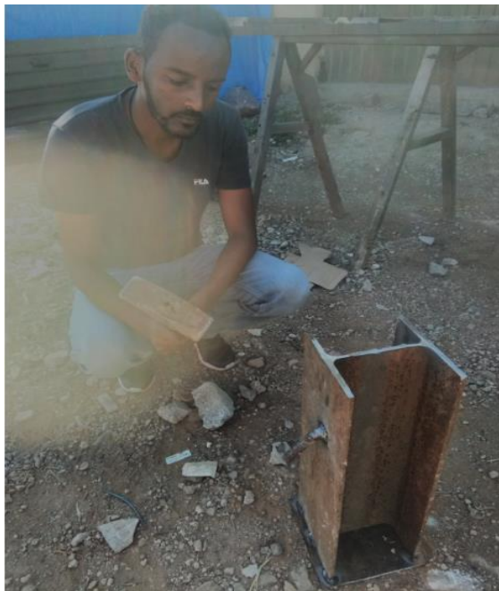
Fig 6.1): performing bend test (To ensure the quality of welding)
