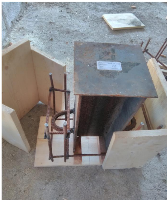
Fig 6.3): formwork preparation for solid concrete
