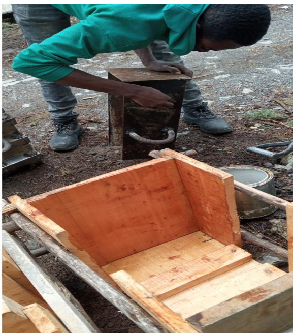
Fig 6.5): oiling the steel and formwork
