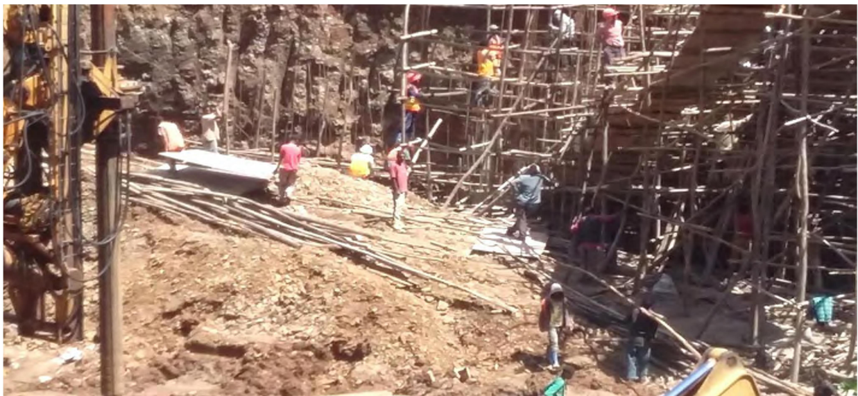
Figure 4.5:- Lack of proper implementation
