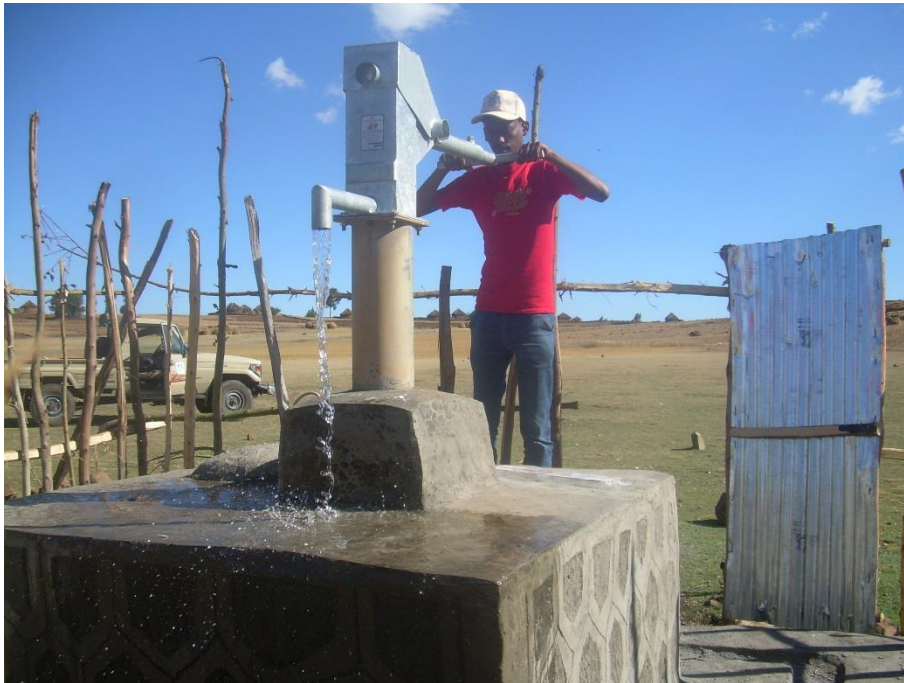
Figure 24-Biret Afer Hand Dug Well with Hand pump
