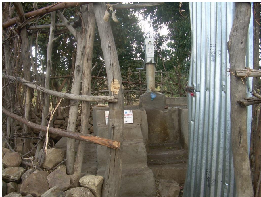
Figure 22-Dens Hand Dug Well with Hand pump
