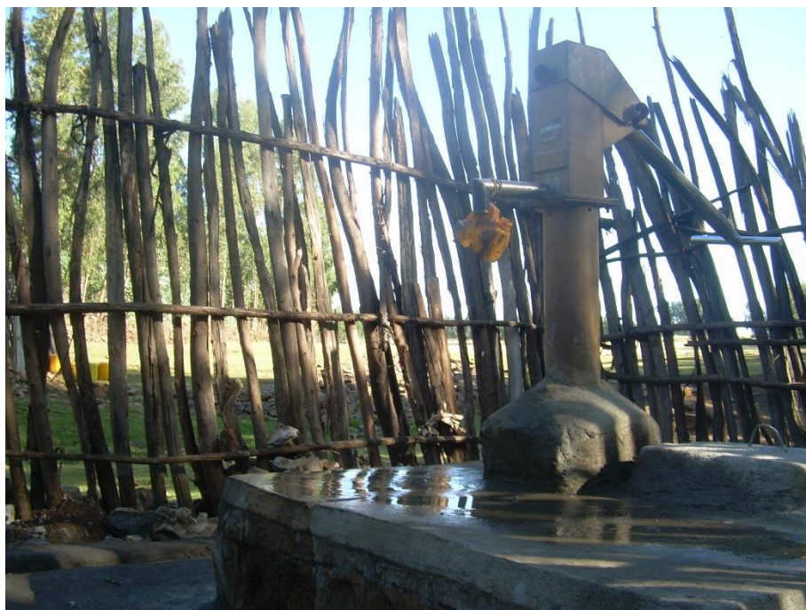
Figure 20-Tunchweha Hand Dug Well with Hand pump
