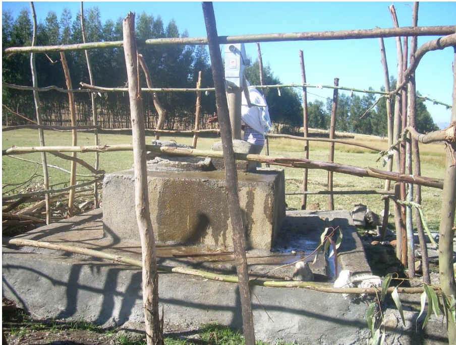
Figure 19-Dirfo Hand Dug Well with Hand pump
