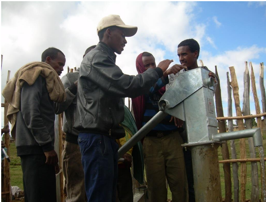
Figure 23-Boya Hand Dug Well with Hand pump
