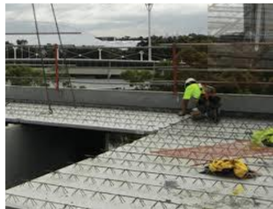
d) Erection of precast lattice plates
