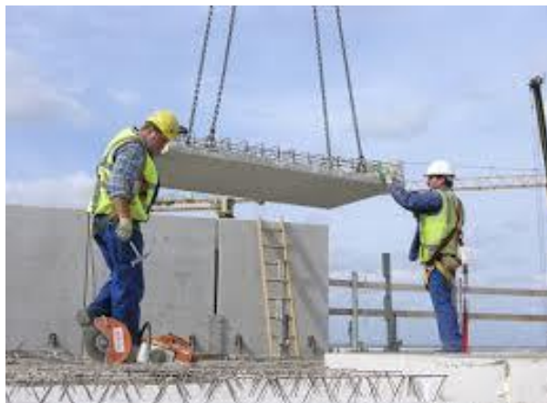
c) Lifting of precast lattice plate
