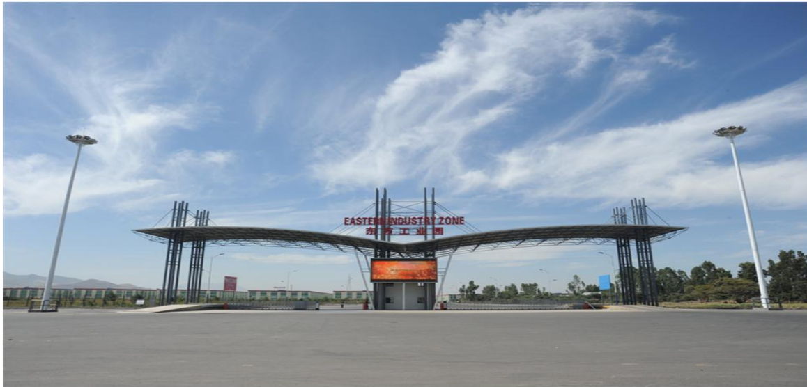
Main Gate of Eastern Industrial Zone
