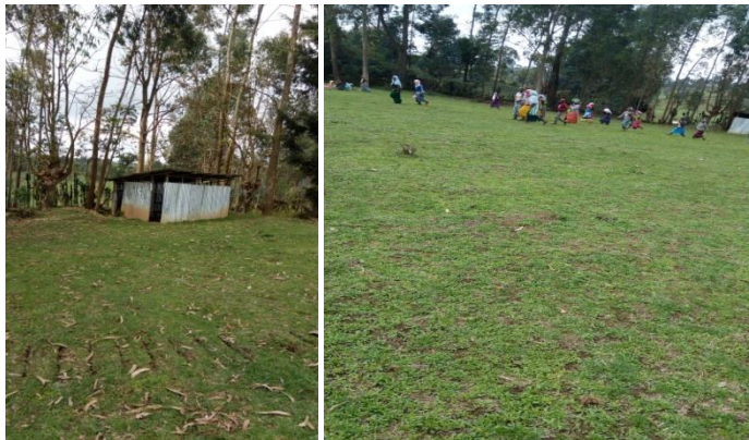
Separate latrine for female students established after the intervention of SAP
