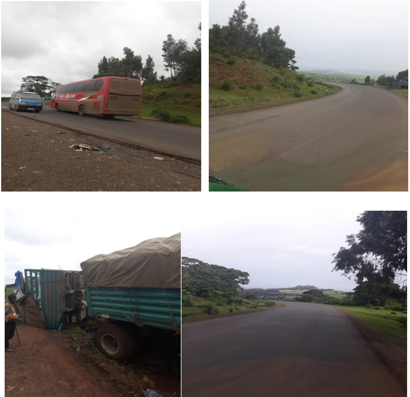
Figure 4.19: Photo of Black Spot Location Conditions with Deficient Geometric Design.
