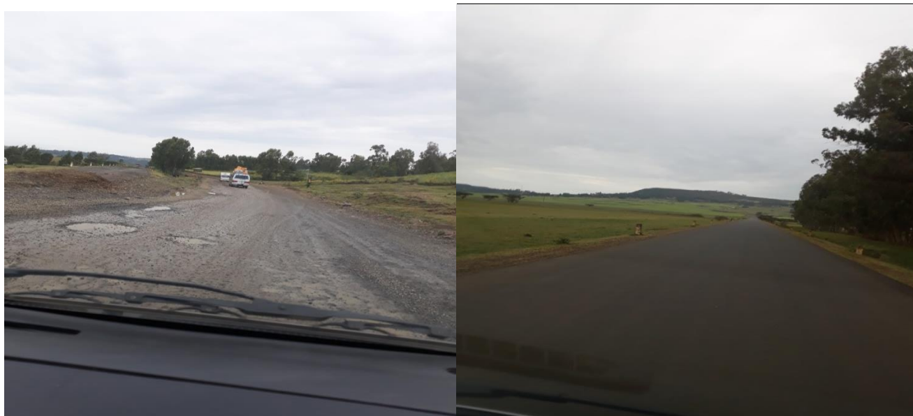
Figure 4.25. Absence of Rehabilitation, Traffic Sign, Pedestrian Crossing and Lane Marking
