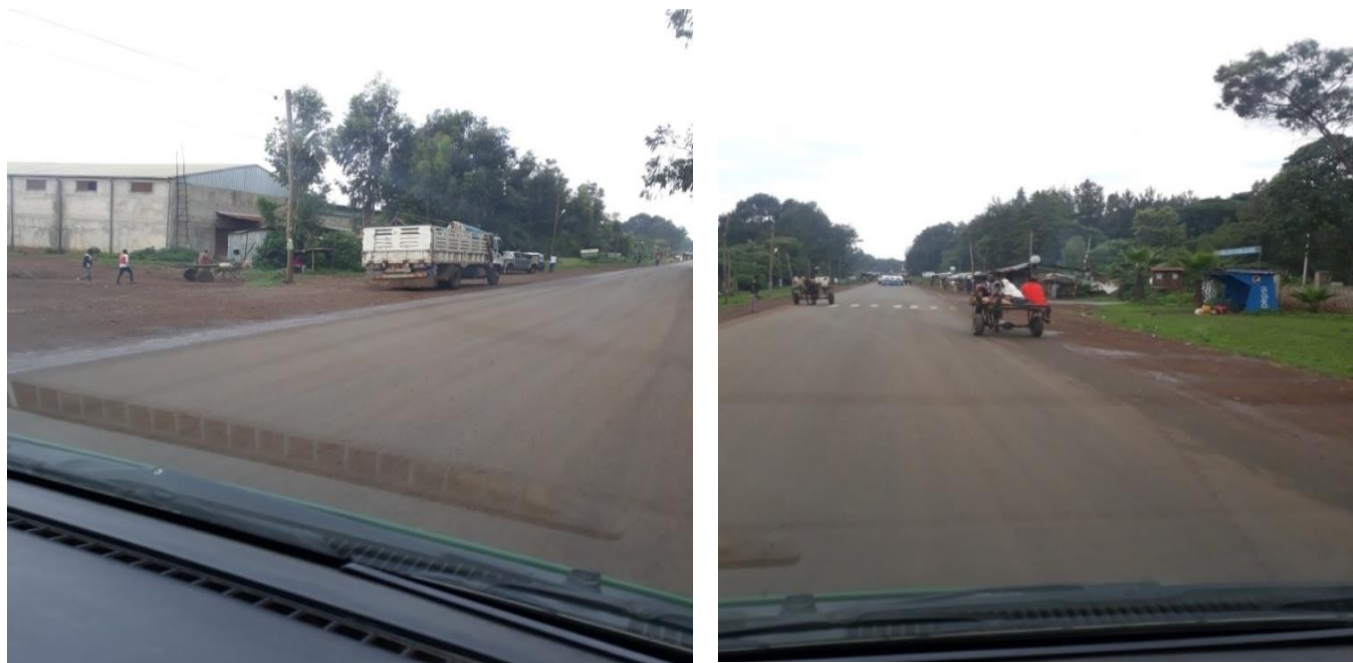
Figure 4.20: Deficient Road Width, Lack of Traffic Sign and Pedestrian Walkway at Burie Town
