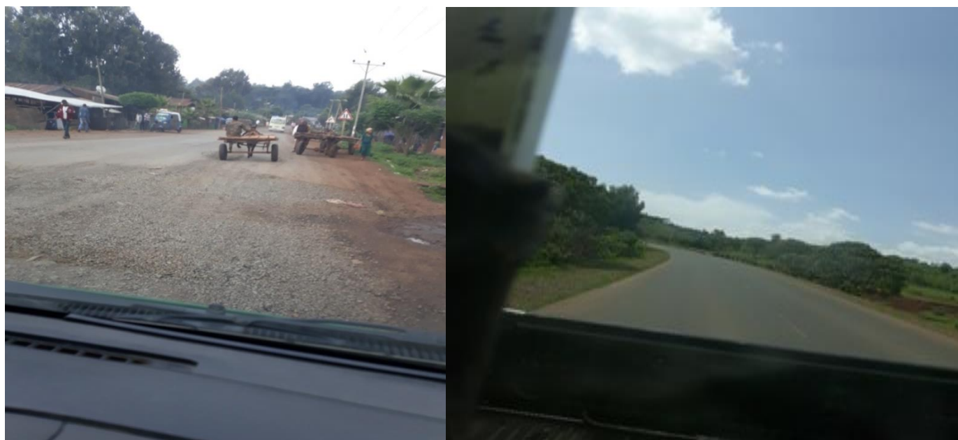
Figure4.21: Photos Showing Lack of Routine Maintenance, Travers and Lane Markings of the Route
