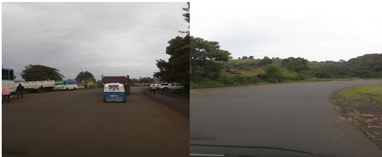
Figure 4.27: Lack of Pedestrian Walkways, Lane and Pedestrian Crossing Marking
