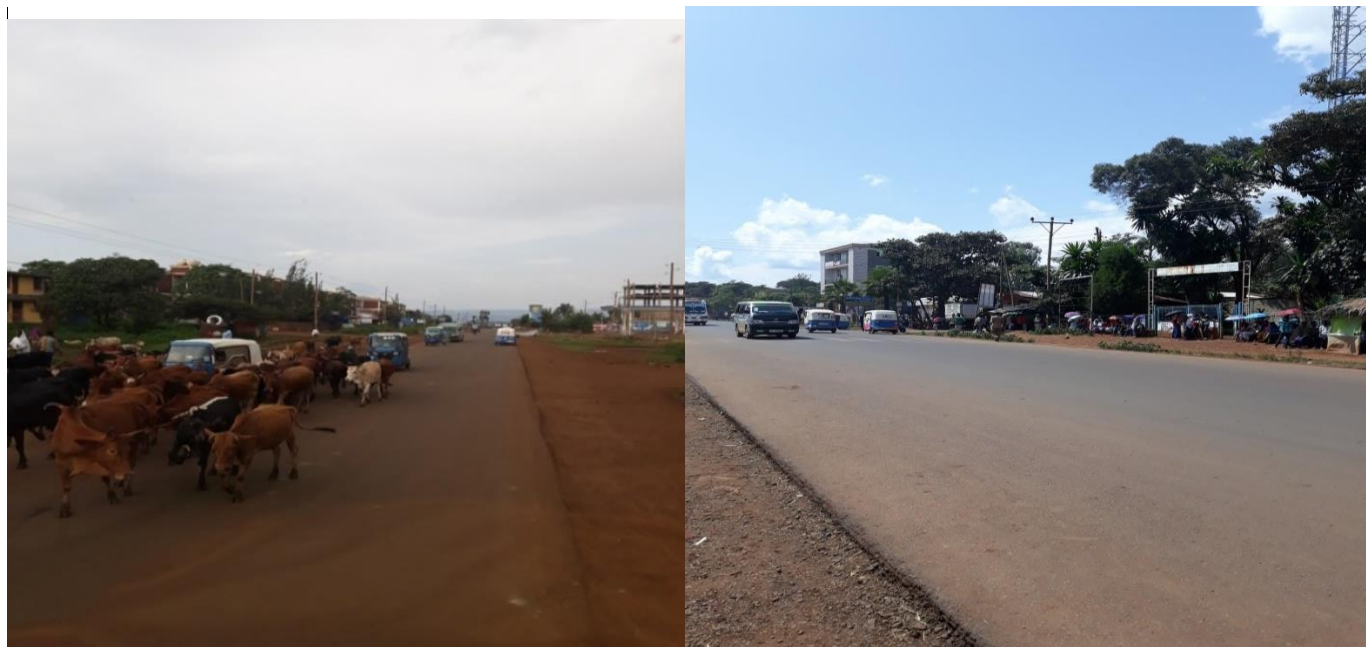
Figure 4.23: Improper Drainages, Lack of Traffic Sign, Pedestrian and Animal Walkways.
