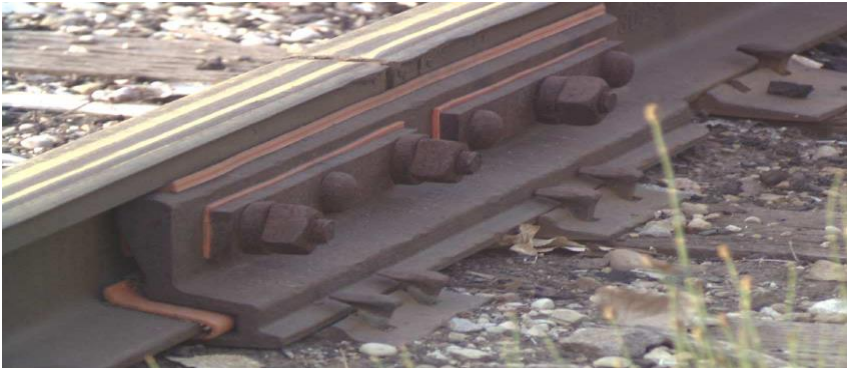
Figure 1.8: Insulated Joints type[29].
