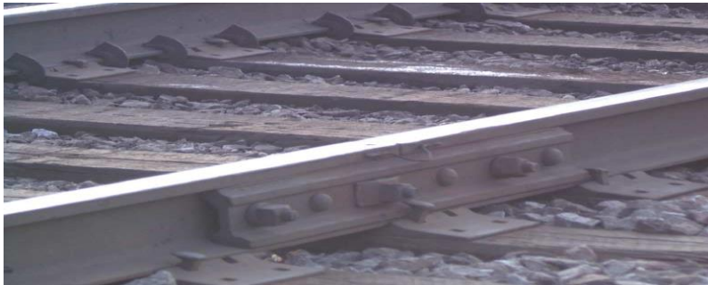
Figure 1.7: Standard Joints[30].
