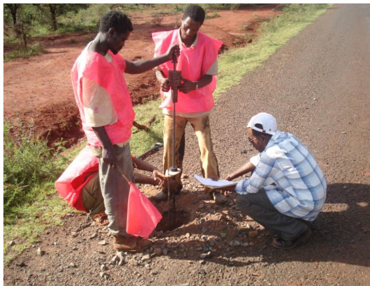
Picture 2.2 Application of DCP in Pavement Investigation (Asphalt Road)
