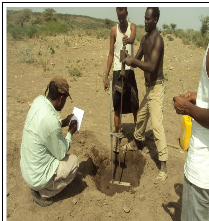
Picture 3.4 Conducting DCP on site (at Sta. 42+500)
