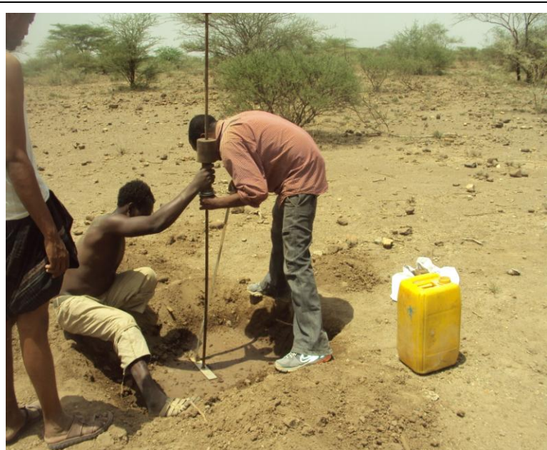
Picture 3.2 DCP Testing Preparation (at Sta. 46+000, C/L)
