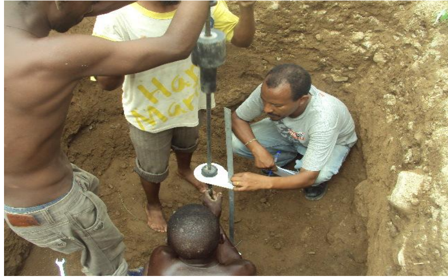
Picture 2.3 Application of DCP in Foundation Investigation (Bridge Structure)
