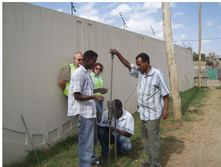
Picture 2.4 Application of DCP in Foundation Investigation (Electric Pole Transmission line)
