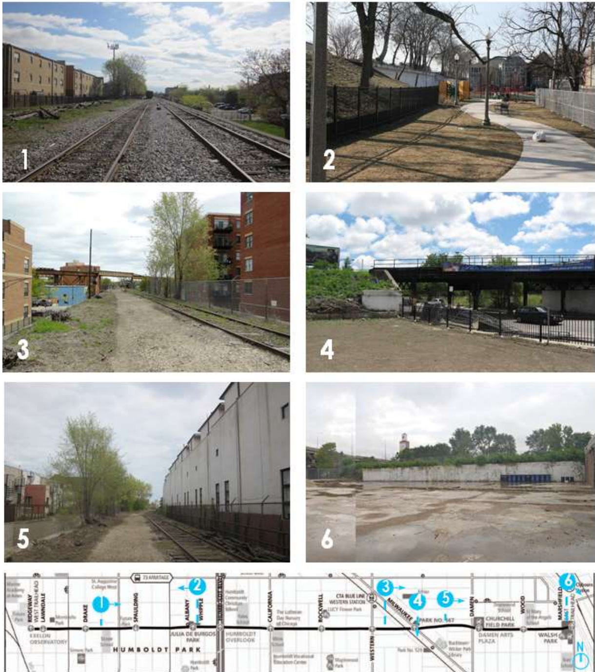
Fig. 38. Site Conditions of The 606 Preconstruction, Source: walking the 606
