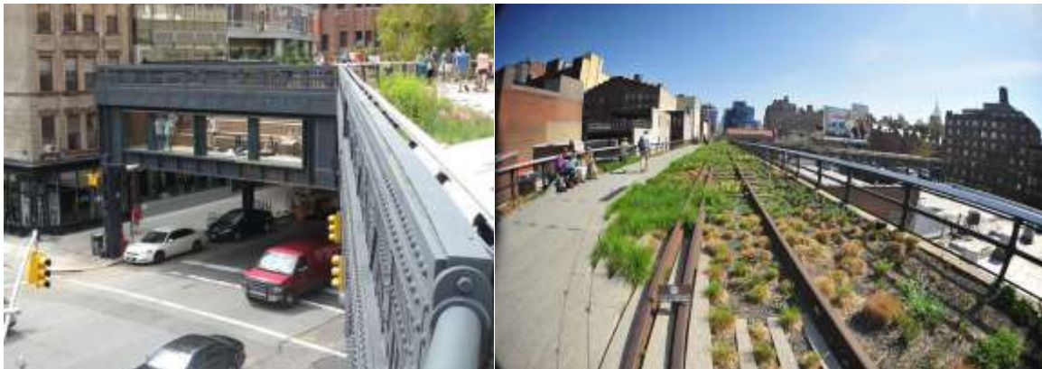
Fig. 13. Art Deco detailing of the rail infrastructure has been restored. Source: www.highline.org
