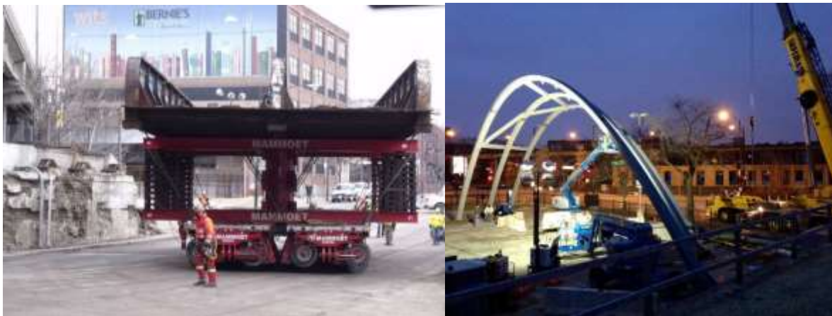
Fig. 43. The structural elements, Source: walking the 606
