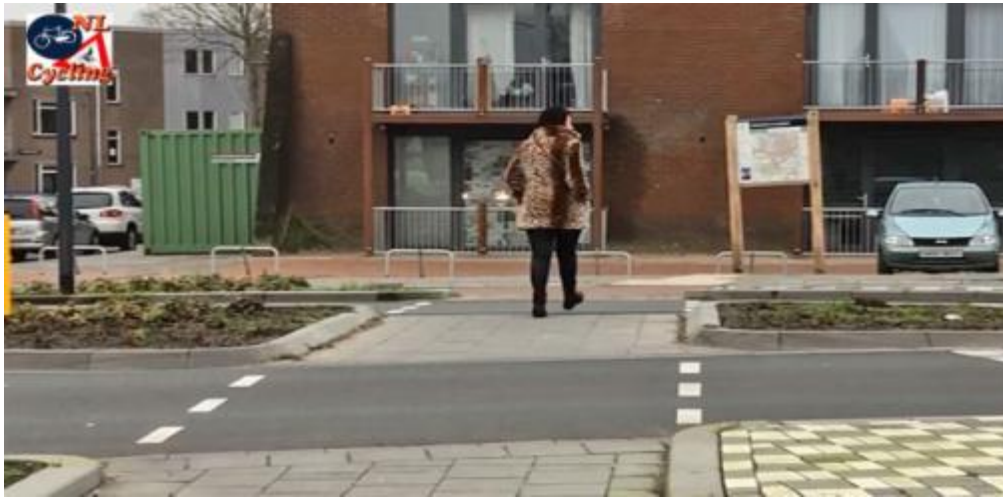
Figure 2.6:- the crossing is flush. There are no kerbs
