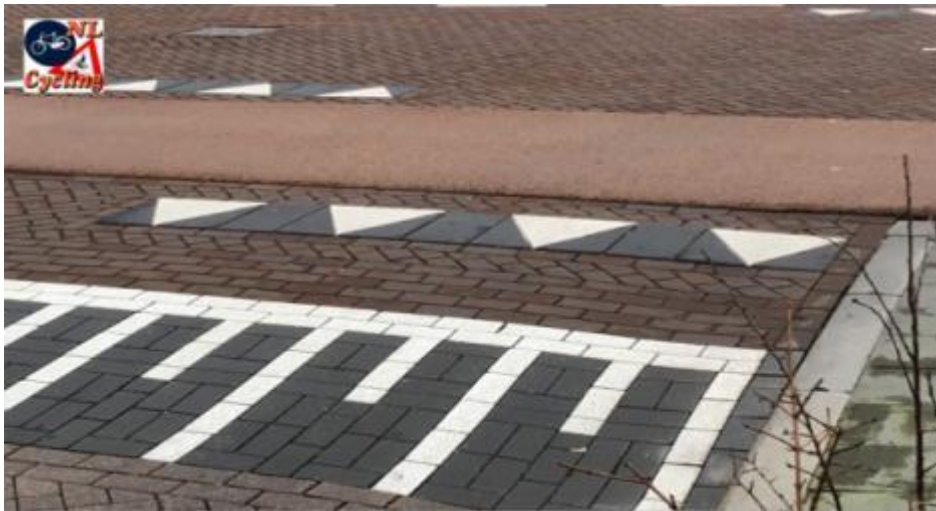
Figure: 2.64 A clear indication of the priority, also in the road surface
