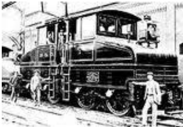
Fig.2.1 The First regular rail service[6]
