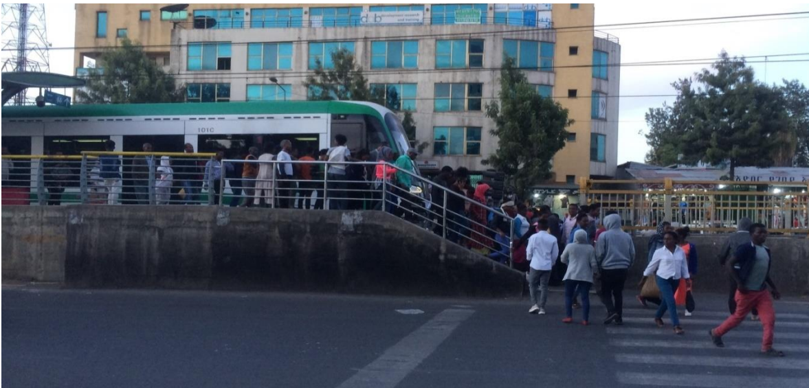
Figure 7: The condition of at-grade pedestrian crossing along AA LRT line at Gurd-Shola station
