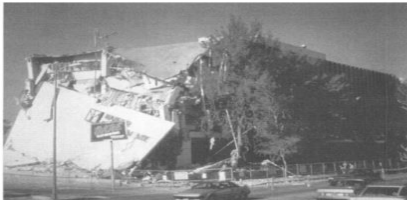
Figure 2: Second story collapse of Kaiser permanent building in Balboa Boulevard at Northridge
