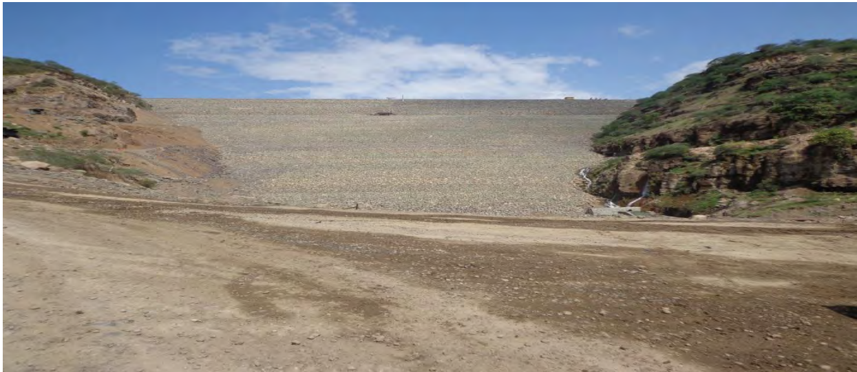
Figure 2.5 Photo of Dam Cross Section Down Stream View
