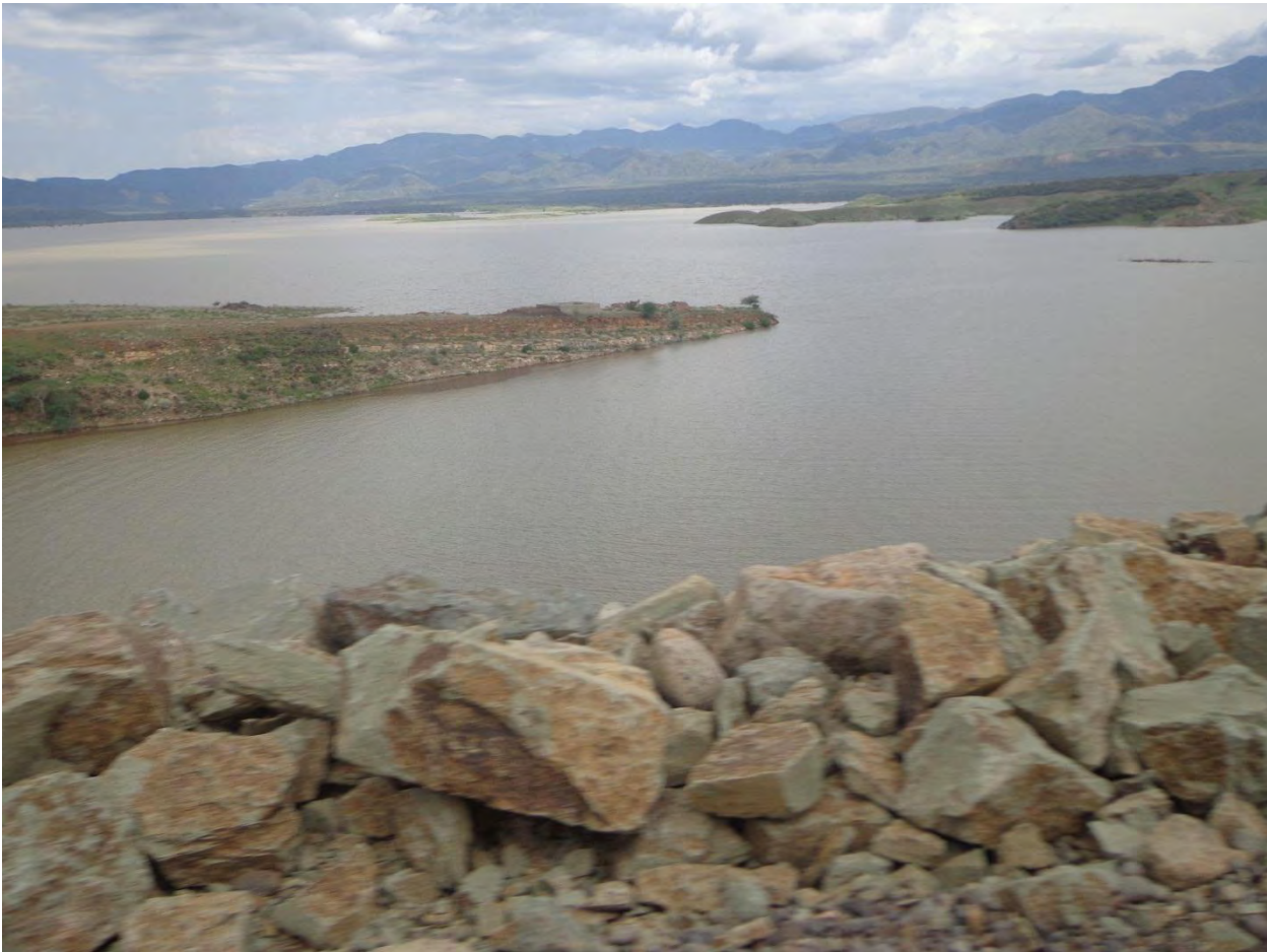
Figure 2.1 Kesem Dam Reservoir
