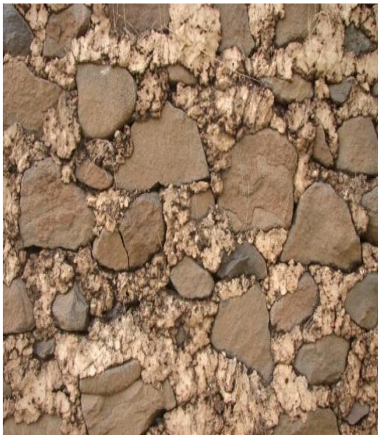
Fig 4.1: Rough Uncoursed Basalt Rocks with White Lime Mortar (Bete Mule, Welkait)
