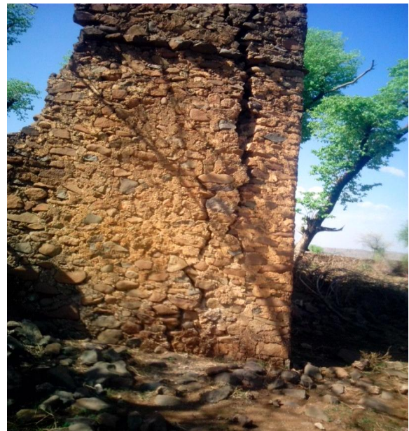
Fig 4.1: Rough Uncoursed Basalt Rocks with White Lime Mortar (Bete Mule, Welkait)
