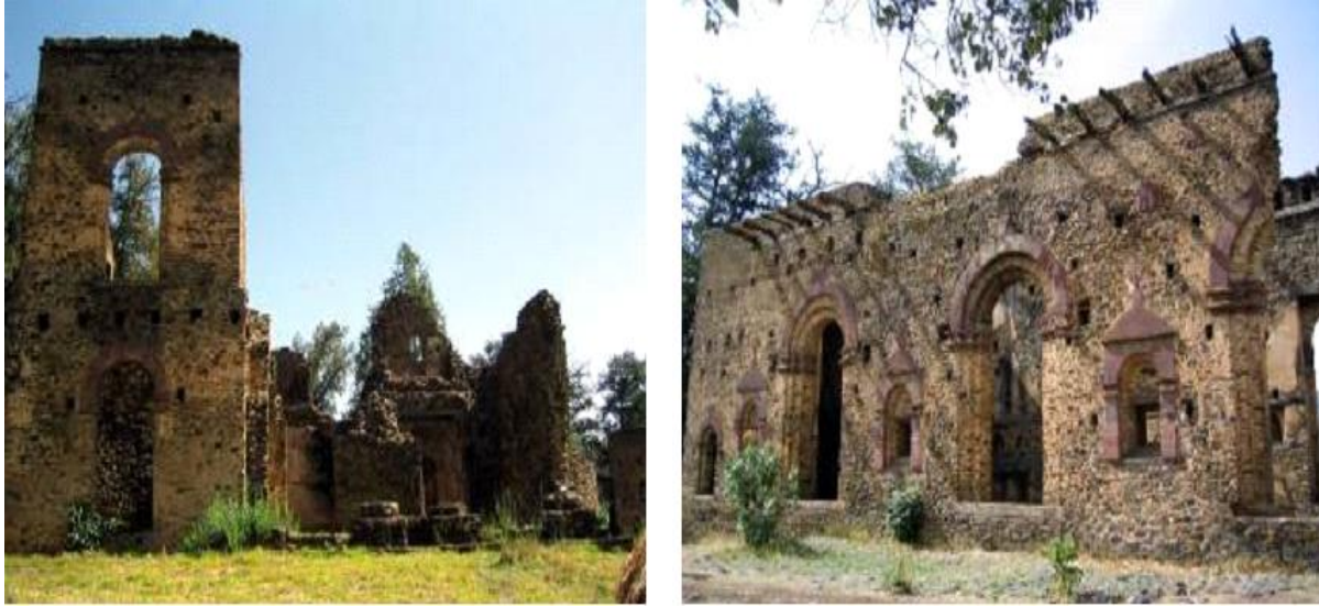
Fig 4.2: Structures of Gondarian Castles (Source: ECHP, 2010)
