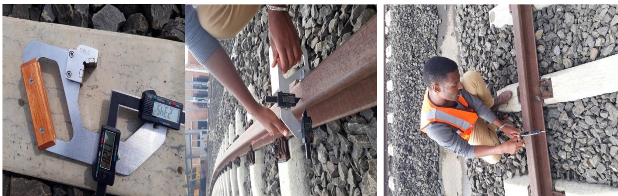
Figure 15: Wear measurement on site
