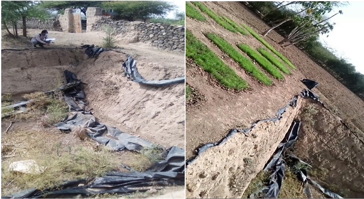
Figure 20: Photos of defected plastic sheet (geo-membrane) usage on ponds
