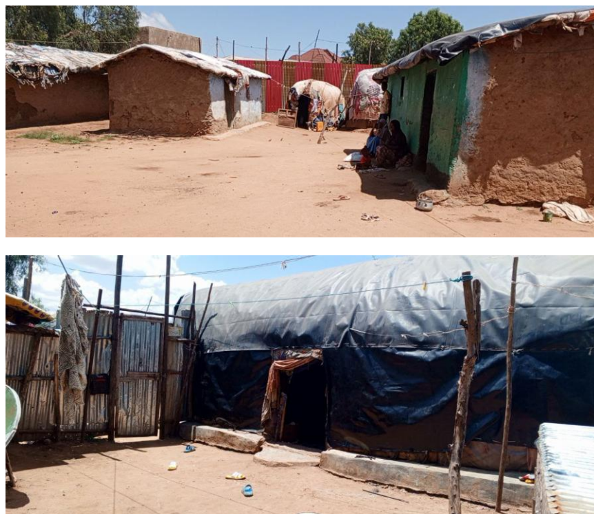
Figure 4.2-46 Shelter Exterior Look
