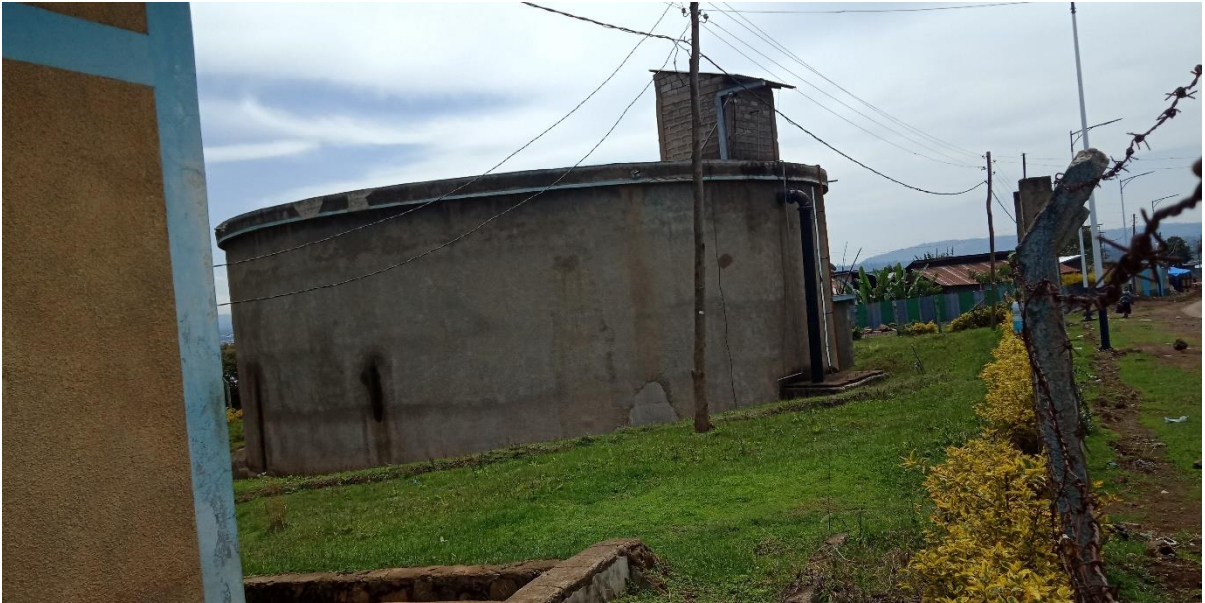
Figure A3: 0:1 Gulit reservoir with 2000m 3 capacity
