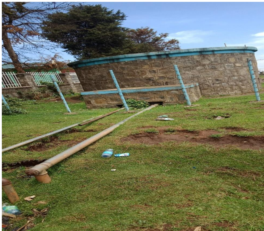
Figure A3: 0:2 Hospital reservoir with 50m 3 capacity
