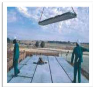
(c) Precast hollow core slabs erected on in-situ beams
