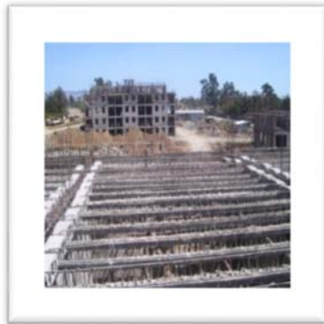
(a) Precast beam installation
