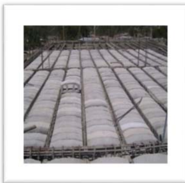
(c) Hollow block installation
