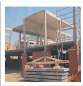
(c) Precast hollow core slabs erected on in-situ beams
