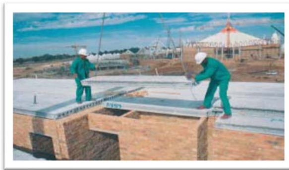
Figure 5.4: Hollow core slab being hoisted into Position.
