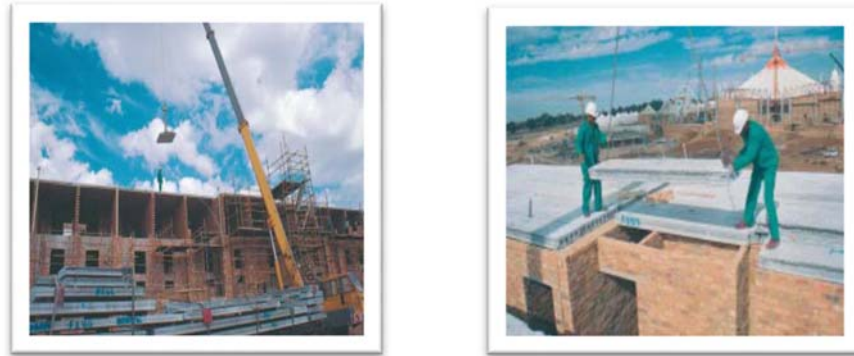
Figure 2.17 Hollow core slabs being hoisted into position by mobile crane
