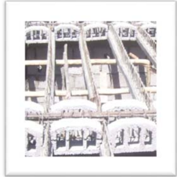
(b) Setting out of hollow blocks
