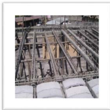
(c) Hollow block installation
