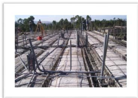
(f) Sanitary and electric conduits Installation
