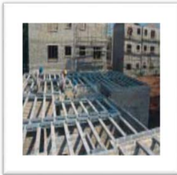
(a) Precast beam installation
