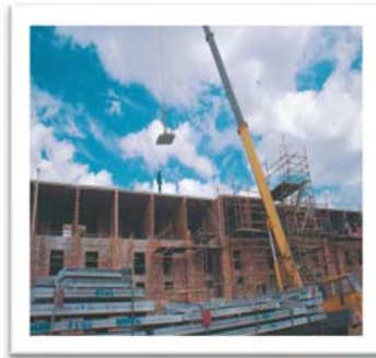
(b) Hoisting hollow core slabs into position
