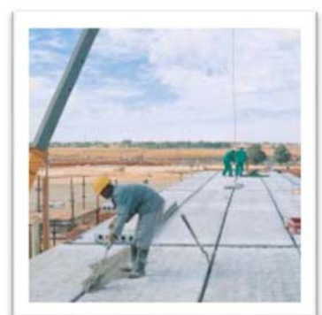
(d) Grouting joint between hollow core slabs
