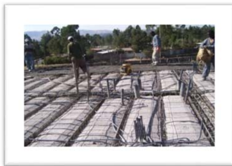
(e) Mesh placed over blocks
