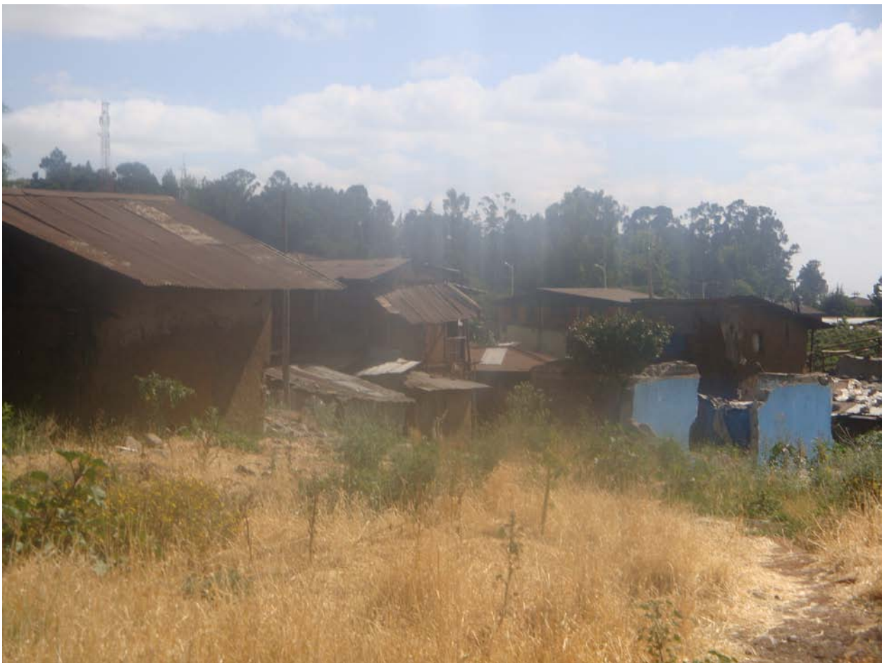
Photo 2: The picture of the largely demolished or almost crumpled area of Basha Wolde II where the remaining 214 residents resided waiting for replacement accommodation or compensation during field study
