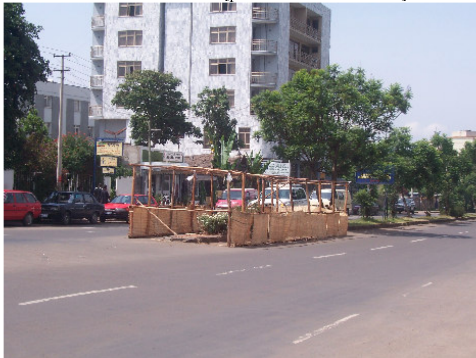
Road barrier covered: [possible cause of collision]
