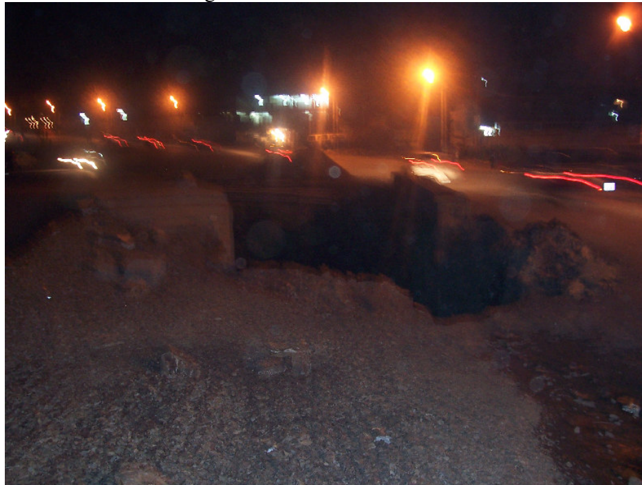
A big ditch in the middle of the road
