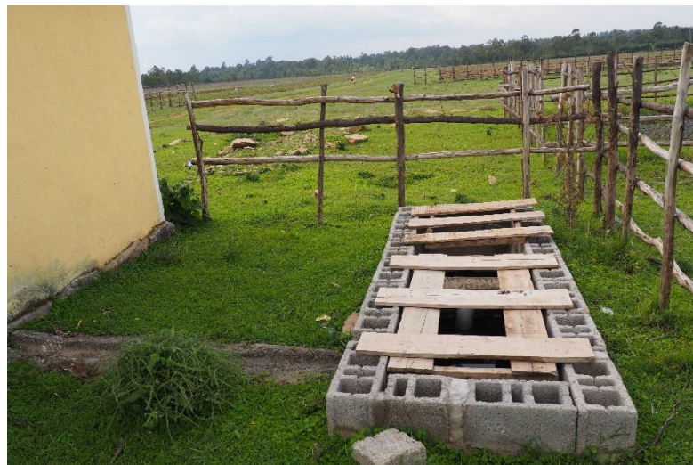
Figure 32wastewater treatment tanks; Photo by the author, June 2019
