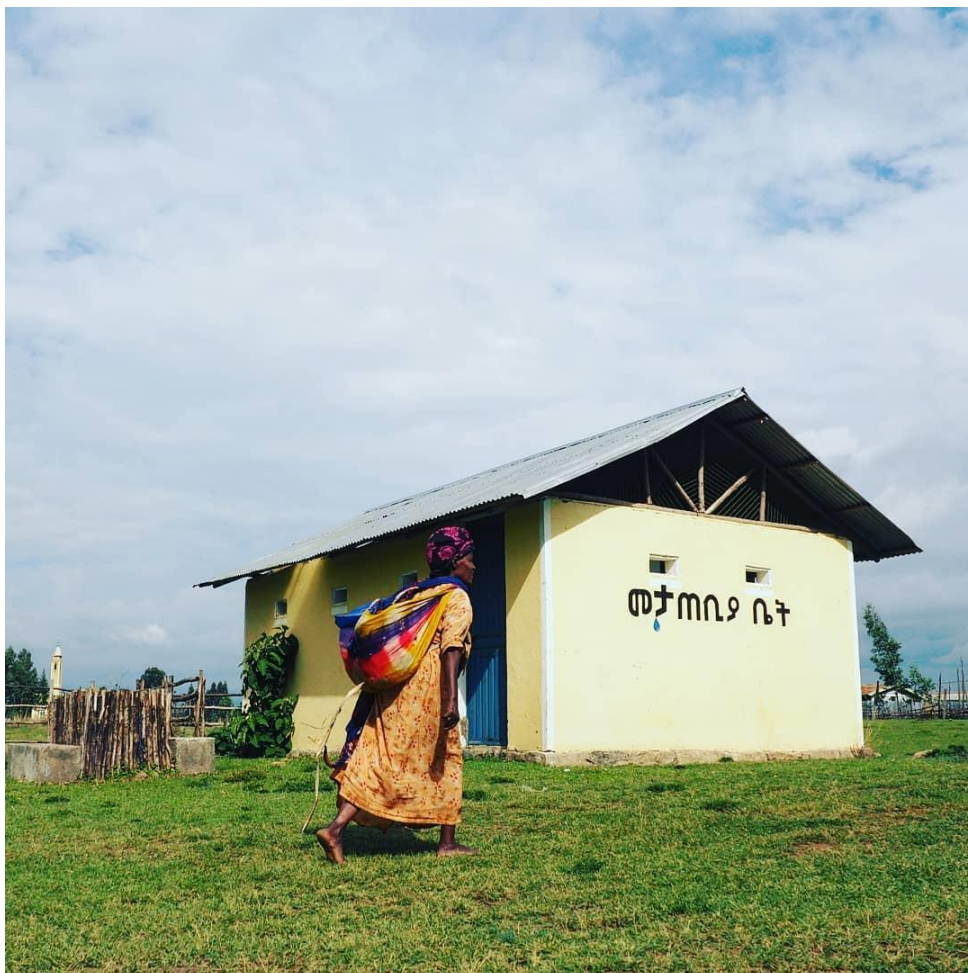
Figure 13 Physical setting and appearance Public sanitation unit in rural context. Photo by Jacob. May2019
