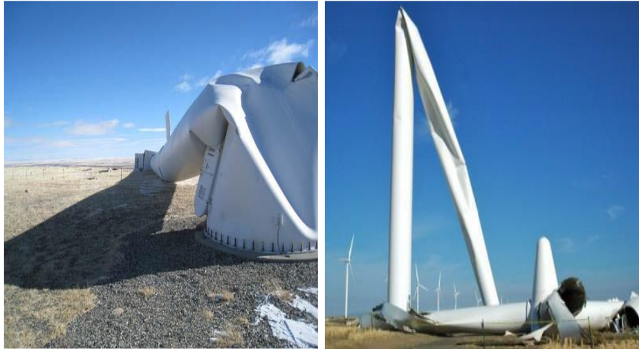
Figure 2.3 (left): Turbine tower failure occurred in Japan
