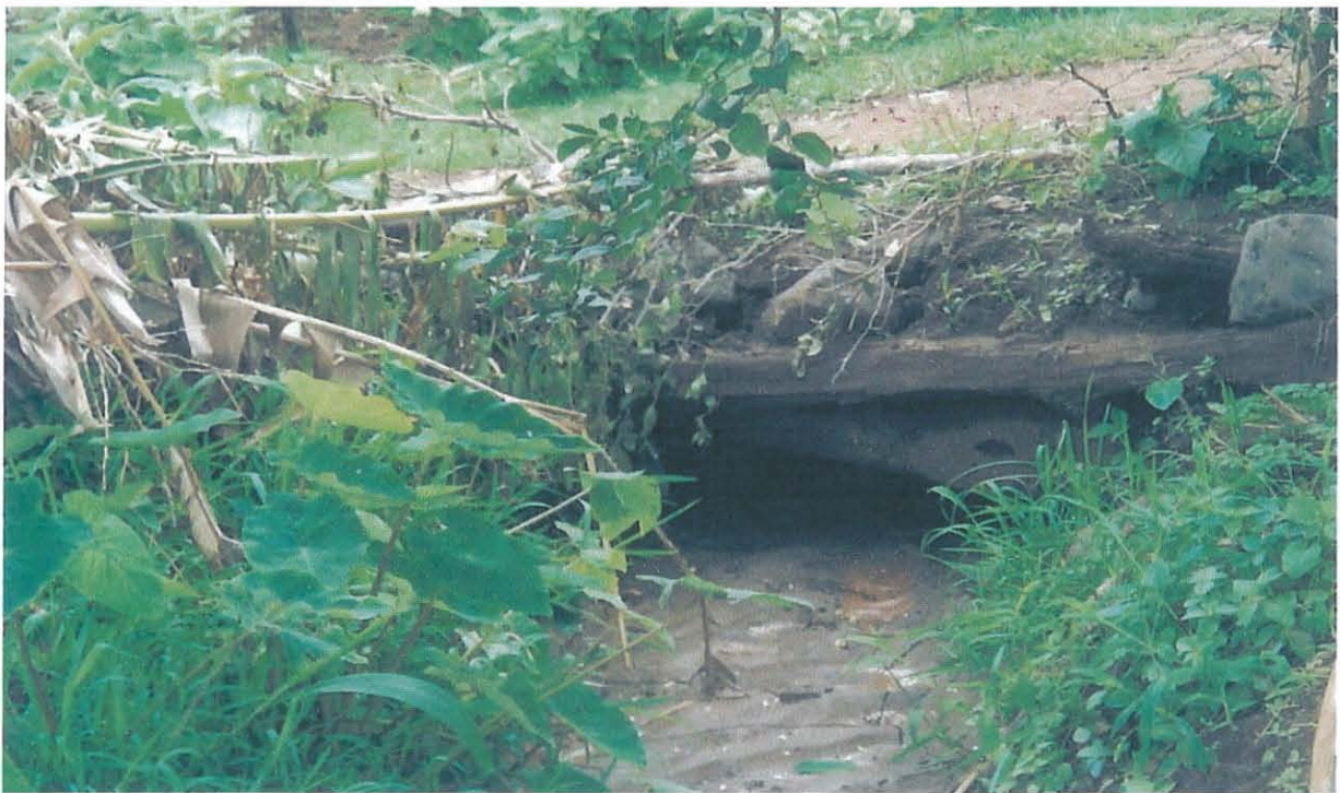
Photo 5.3: Jijolla irrigation head work constructed with wood to carry water to the fields
