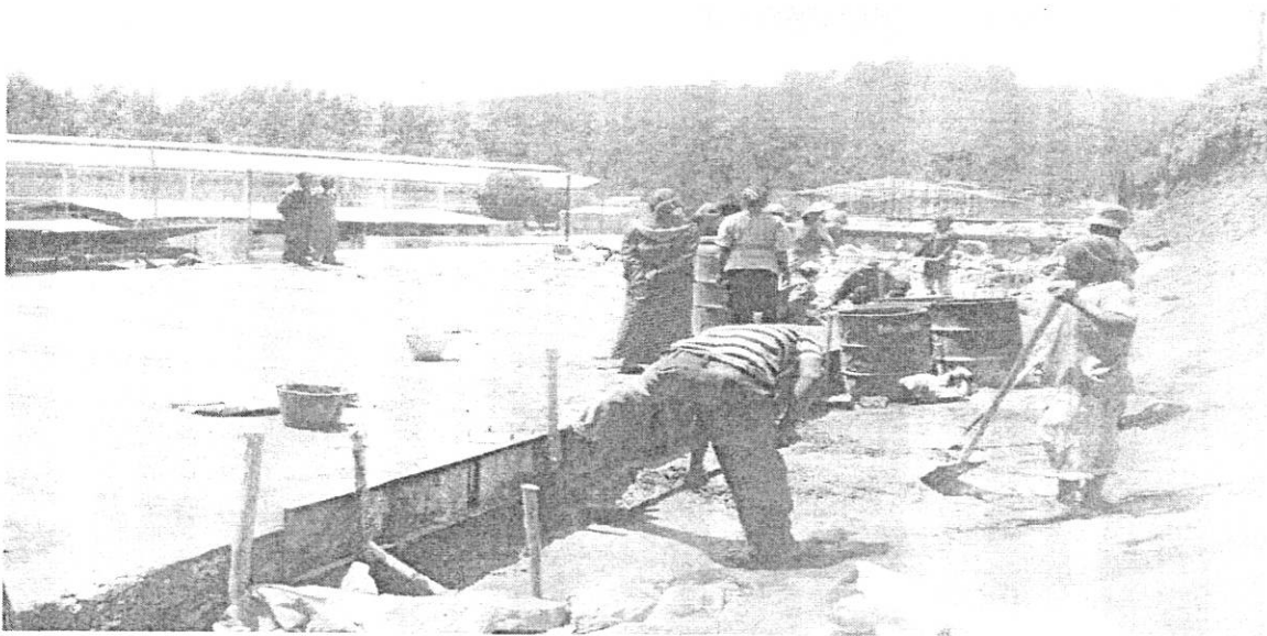
Partial photo view of General Wingate Construction Site
