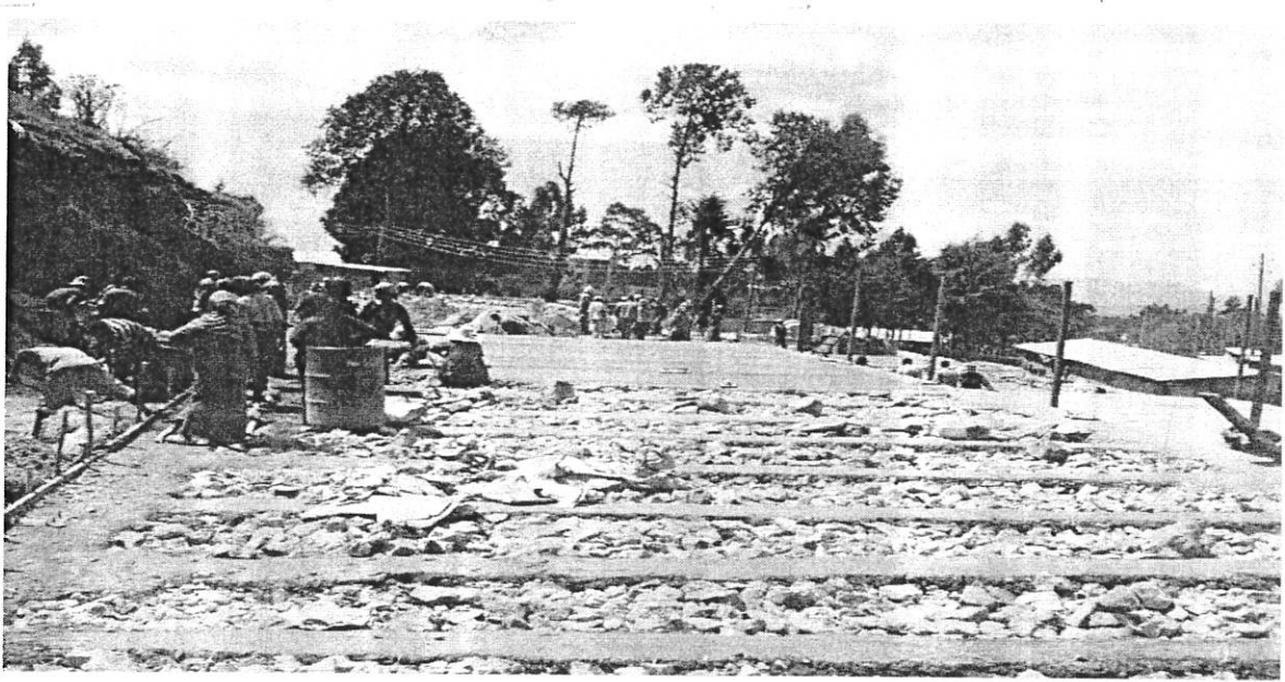
Partial photo view of General Wingate Construction Site
