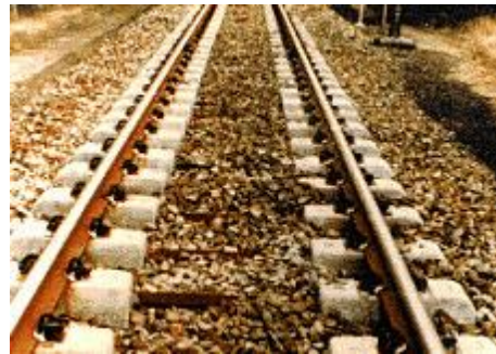
b) Twin-block concrete sleeper
