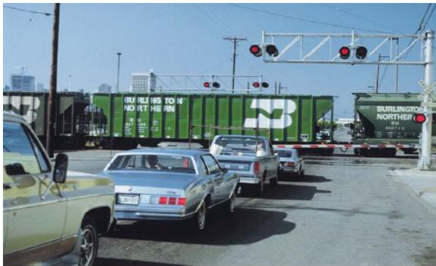
Figure 2.23: highway-railway level crossing safety system [Peterman, 2007]
