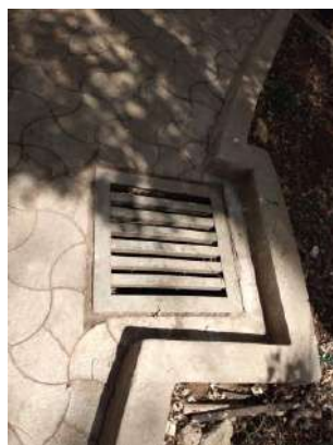
Figure 4.31: Impervious surface with drainage line
