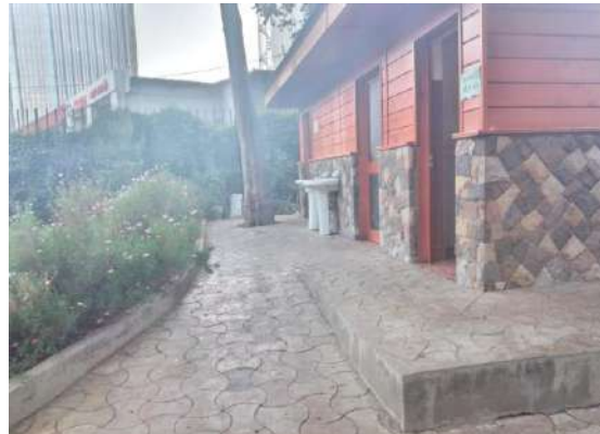
Figure 4.10: Ramp Access for wheelchair
