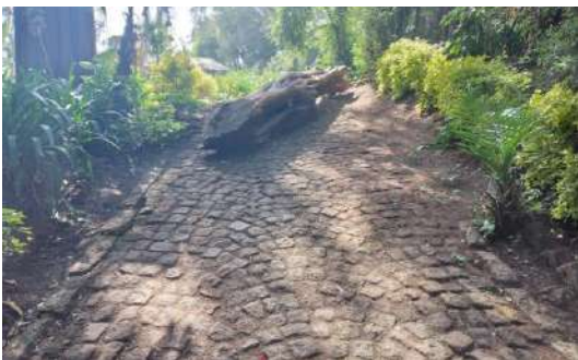
Figure 4.81: Bumpy cobble walkways blocked by tree trunk
