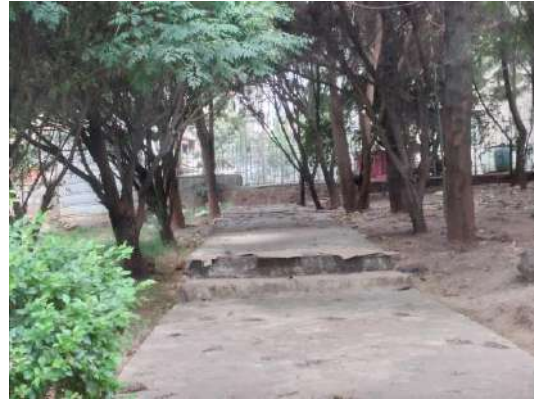
Figure 4.43: Pedestrian step asphalt path
