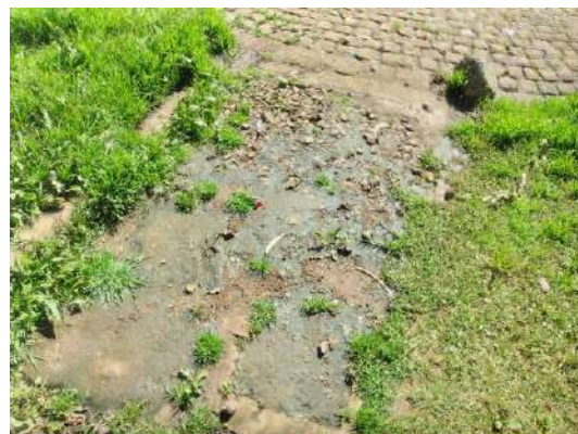
Figure 4.102: sewerage residual creates algae and insect breeding surface
