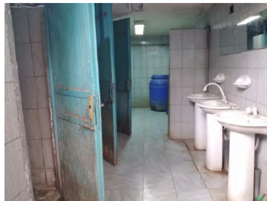
Figure 4.53: Toilet indoor space with hand wash and seat
