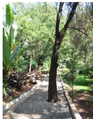
Figure 4.84 Tree obstruct walkways
