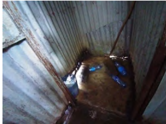
Figure 4.91: Dirt toilet indoor space
