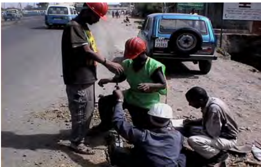
Figure 3.4 DCP Surveys on Test Road No 1
