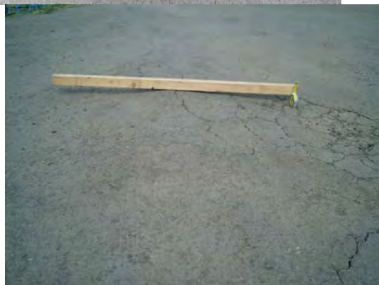
Figure 2.19 Slippage cracks
