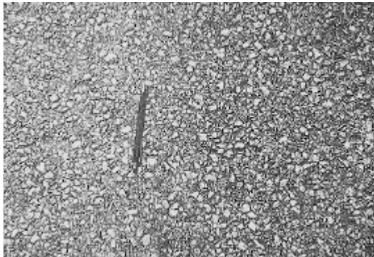
Figure 2.11 Longitudinal crack patching
