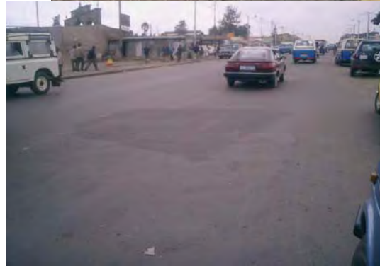
Figure 2.11 Longitudinal crack patching
