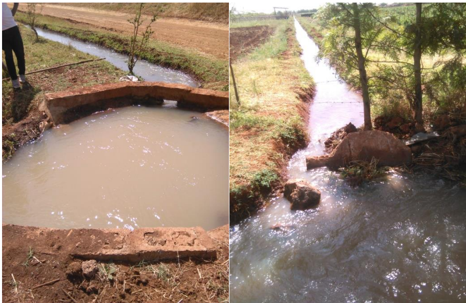
Figure 13 Water delivery structures at tertiary canal
