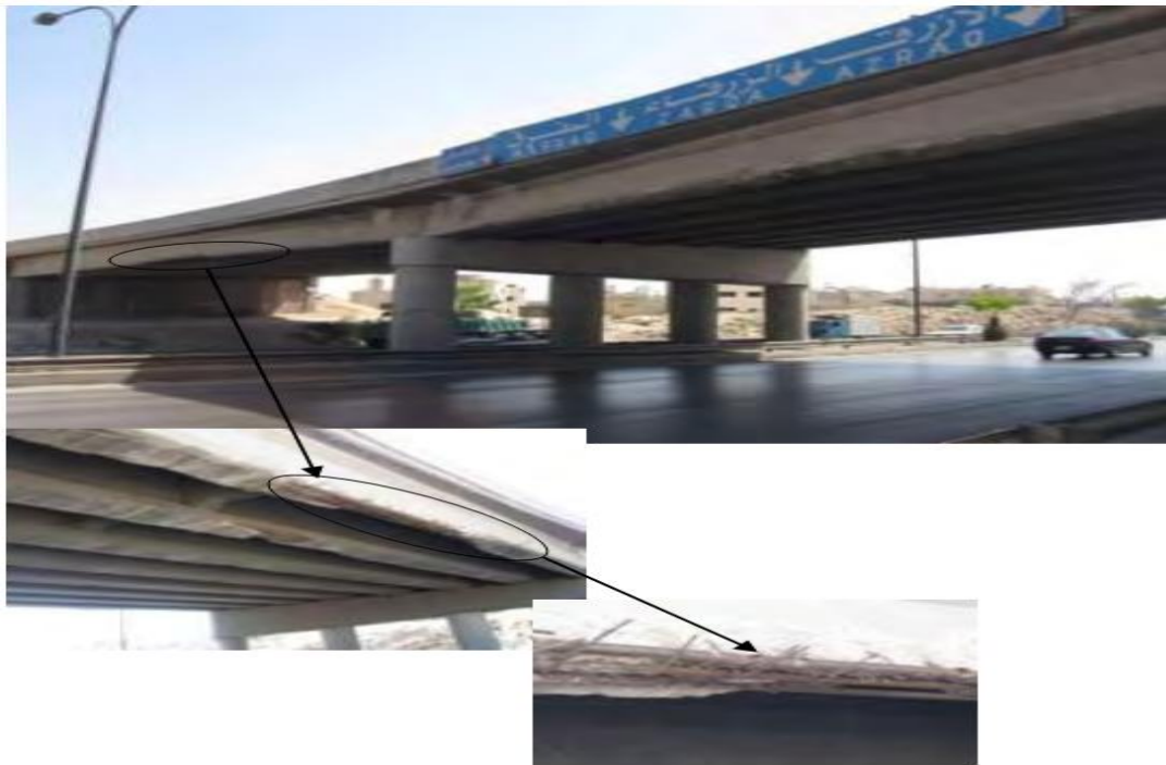
Figure 1 Bridge in the Al Zarqa-Jordan.
