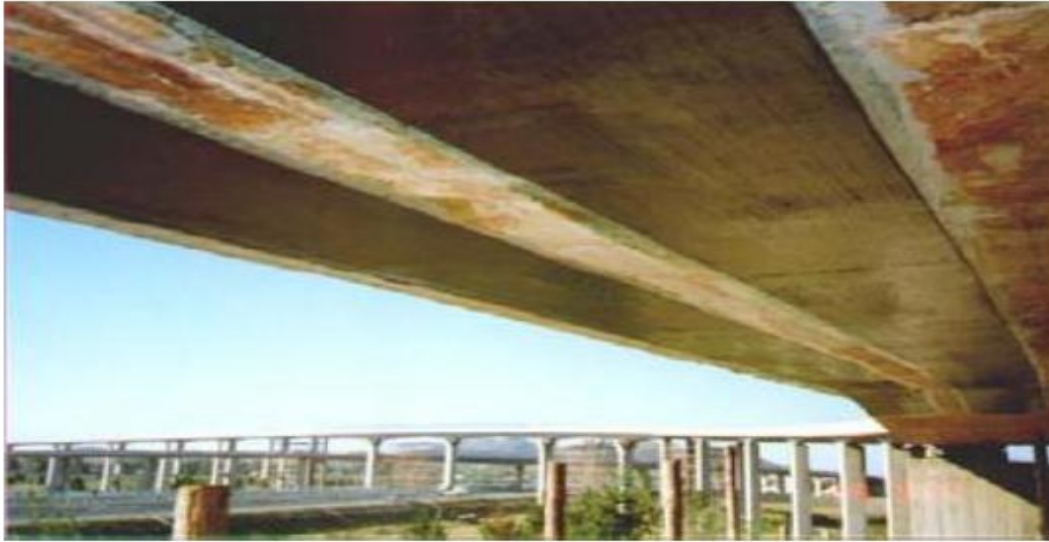
(a) Flexural strengthening of a highway RC bridge slab in China.
